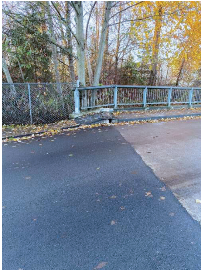
Photograph 8 – Lucille Starr Bridge – west end of bridge looking south; notable separation between bridge and sidewalk.
