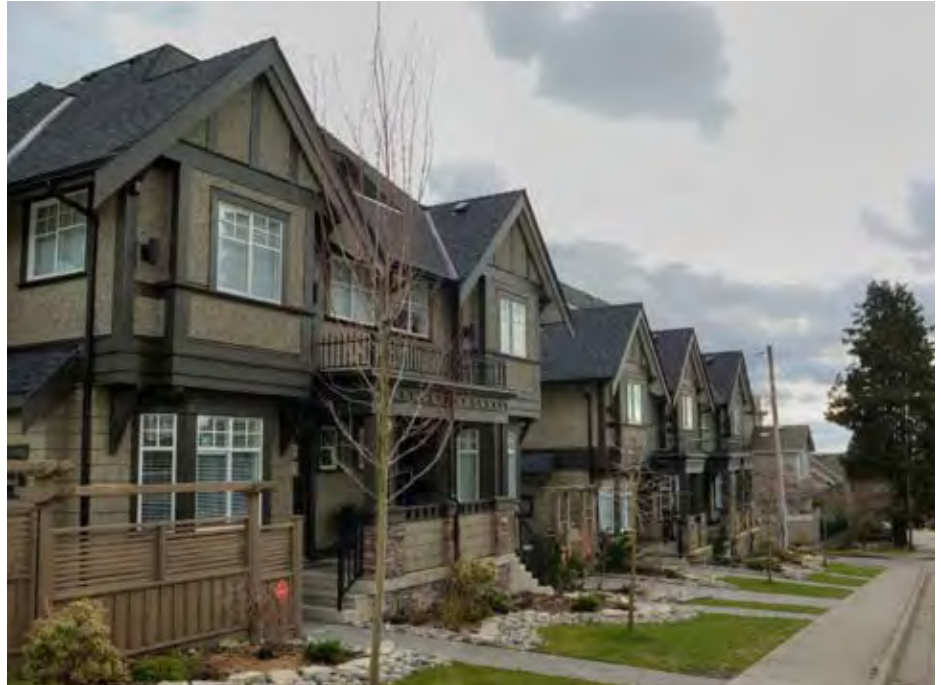
Units stepping down slope along St. George's Avenue
