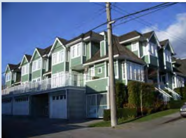
On-grade parking on lane
