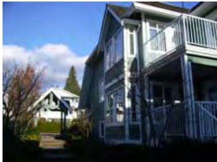
View from courtyard
