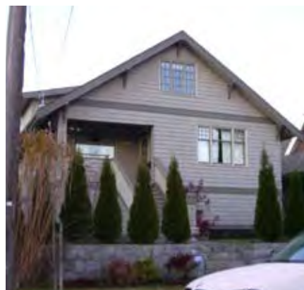
East 12th streetscape - principal house
