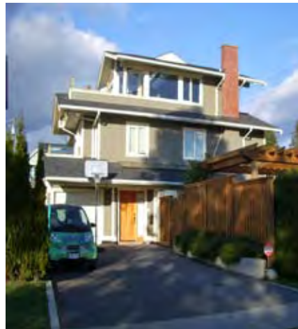
Renovated duplex facing East 9th Street
