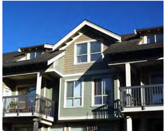
Top floor has living space within the roof structure
