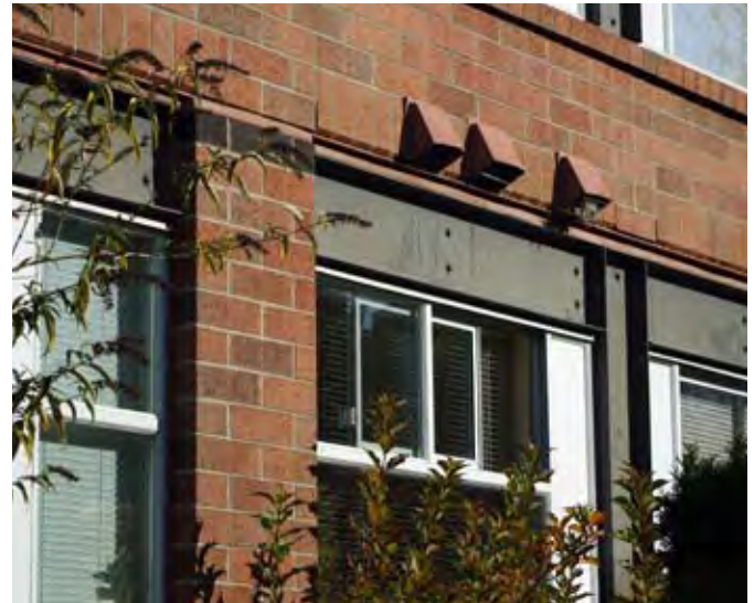
Steel girders become a design feature
