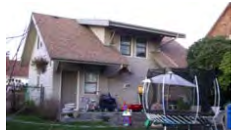
Front elevation of coach house
