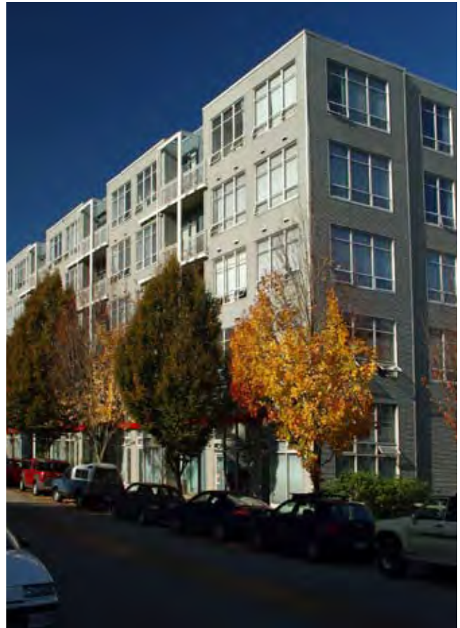
Building materials reflect neighbourhood character
