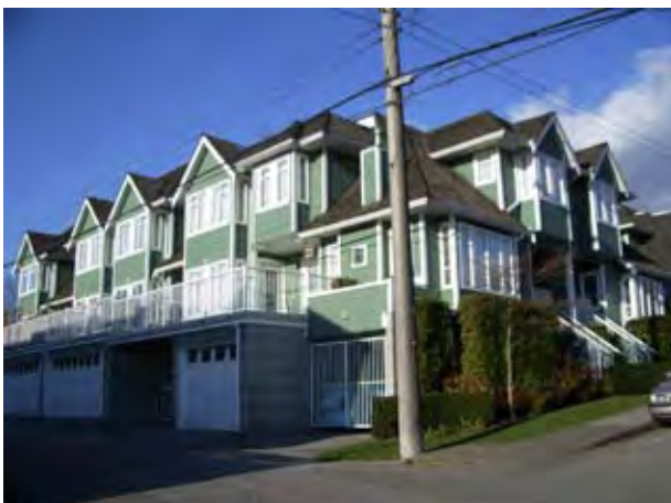
On-grade parking on lane
