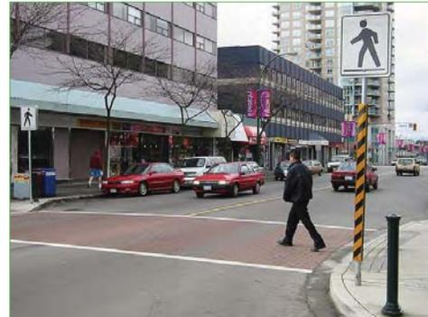
*Sample curb extension at a crosswalk to reduce road width and increase visibility.*
