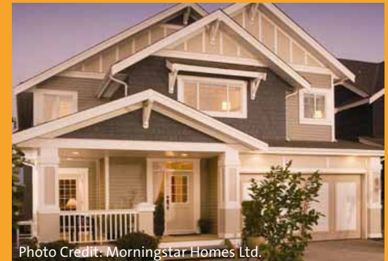
Photo Credit: Morningstar Homes Ltd.
