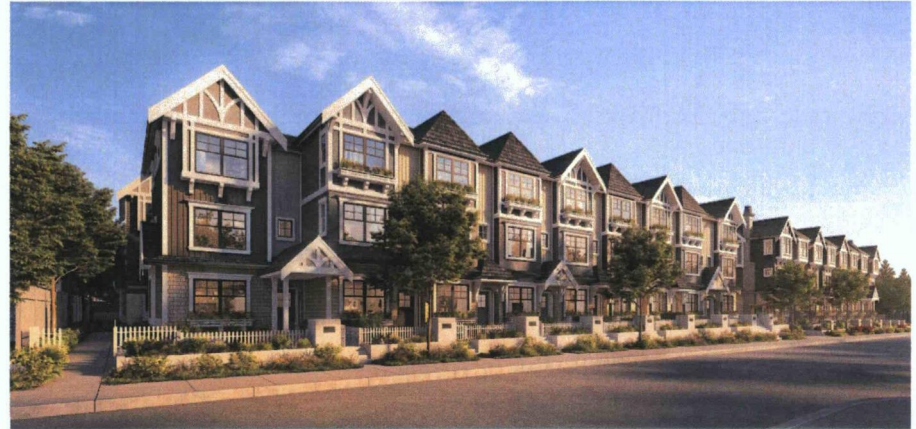
The Robinsons Coquitlam, BC Homes: 34 Lock-Off Units: 8 Under Construction
