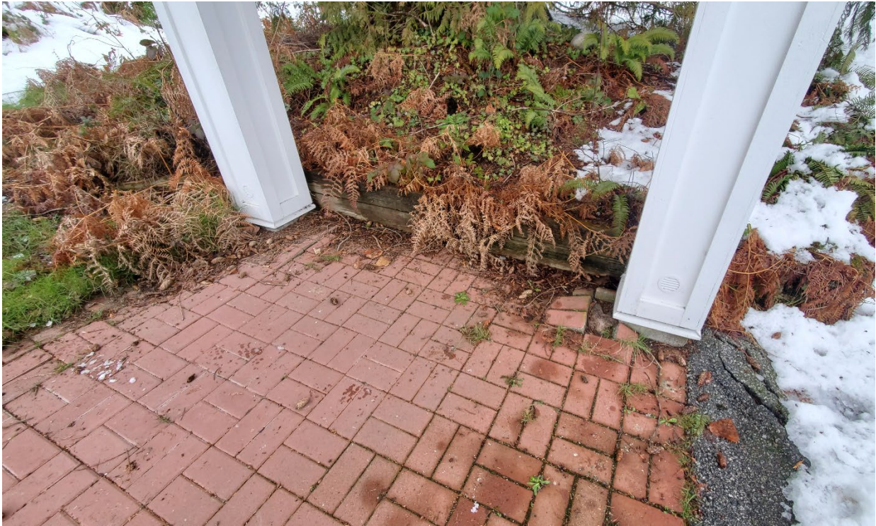
Photo 6. C24 and C25 roots lifting asphalt and brick walkway.
