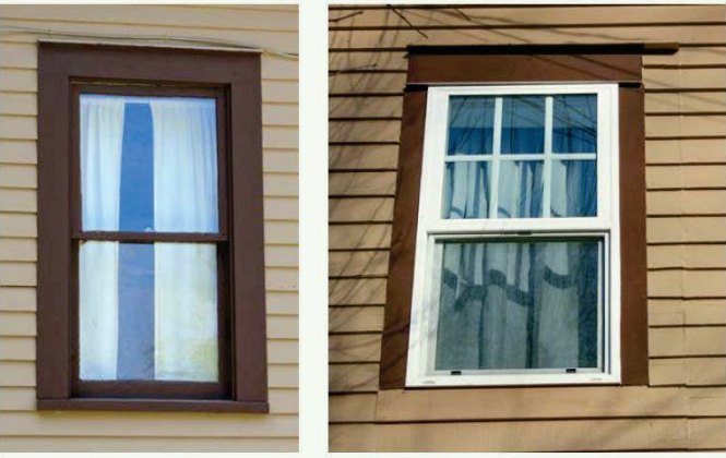
Example of an original wood sash window (left, 2022), and a modern replacement within a resized original window opening (right, 2024), Luxton Heritage
