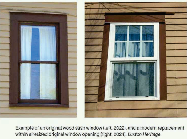
Example of an original wood sash window (left, 2022), and a modern replacement within a restored original window opening (right, 2024), Luxton Heritage
