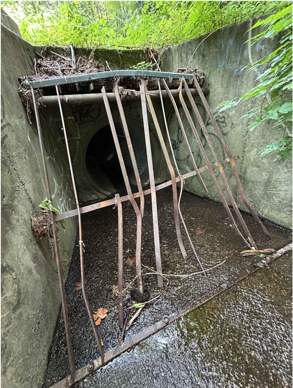
PHOTO 1: EXISTING DEBRIS SCREEN
