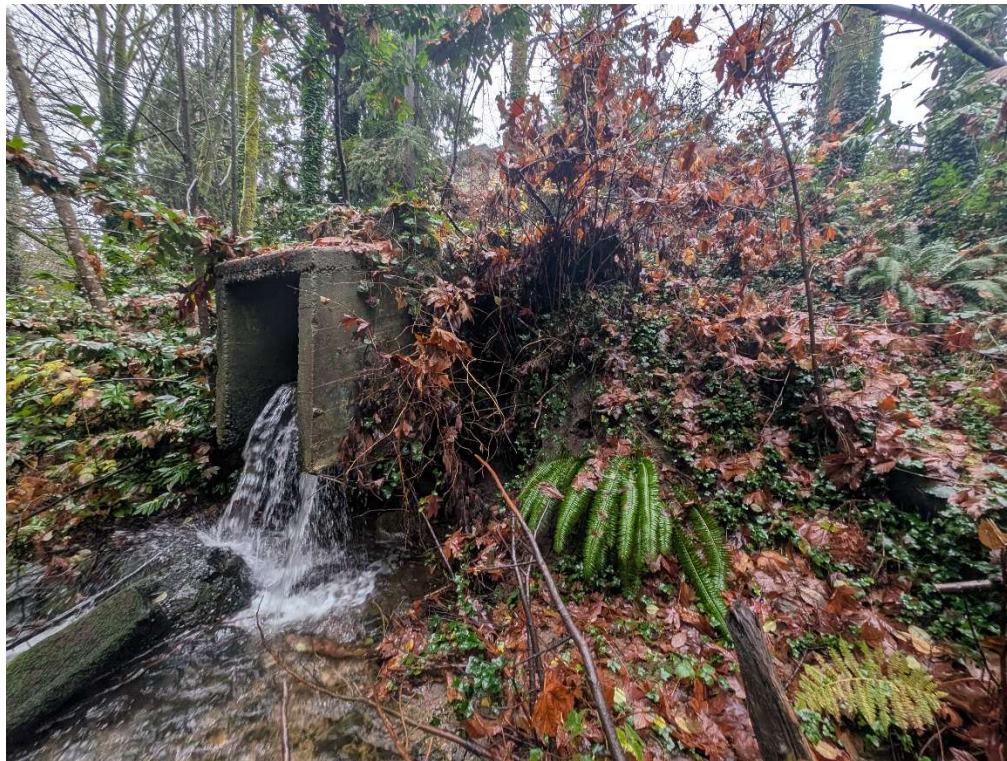
Photograph 2 – Overview of the outfall (Looking north).
