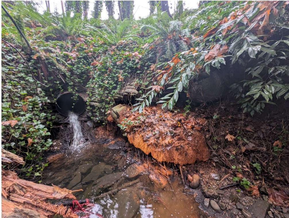
Photograph 1 – Overview of the outfall (Looking northwest).
