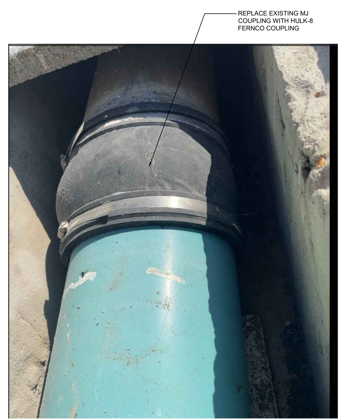
2 EXISTING SUPPLY PIPE SCALE: NTS
