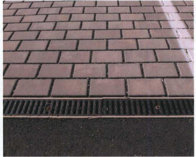
Fig.80 Permeable paving in a parking lot
