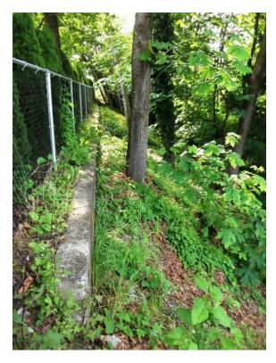
Photo 4: View along City concrete retaining wall above debris flow headscarp and below Corona Crescent. The wall is generally straight.
