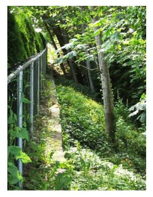
Photo 5: View along City concrete retaining wall with outward bulge, west along Corona Crescent from headscarp area. Small deciduous trees have tipped from shifted surface soils.
