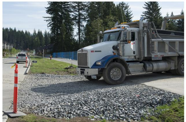
Rock mulch pads require frequent inspection and repair/replacement to maintain their function and preclude offsite tracking.
