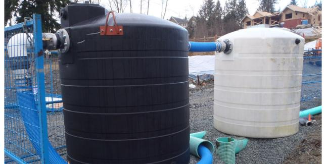
Portable tanks may also provide suitable detention in support of localized dewatering requirements where discharge to the municipal storm system or watercourses would be prohibited due to turbidity levels.
