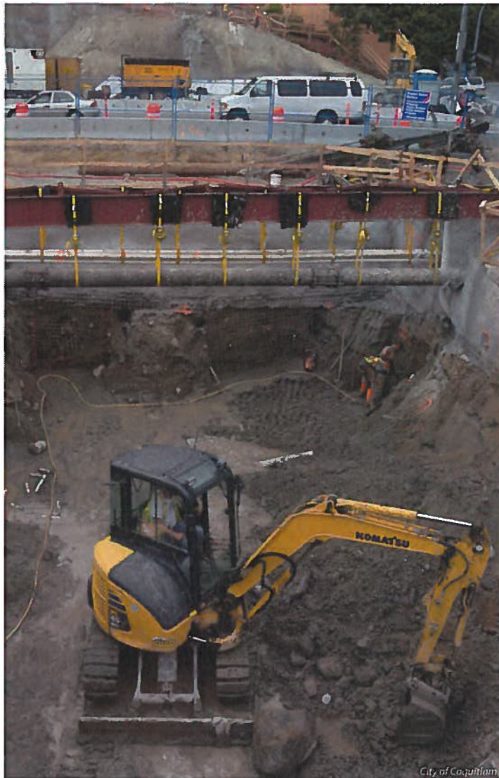
City of Coquitlam Tunnel being constructed under the Barnet Highway.
